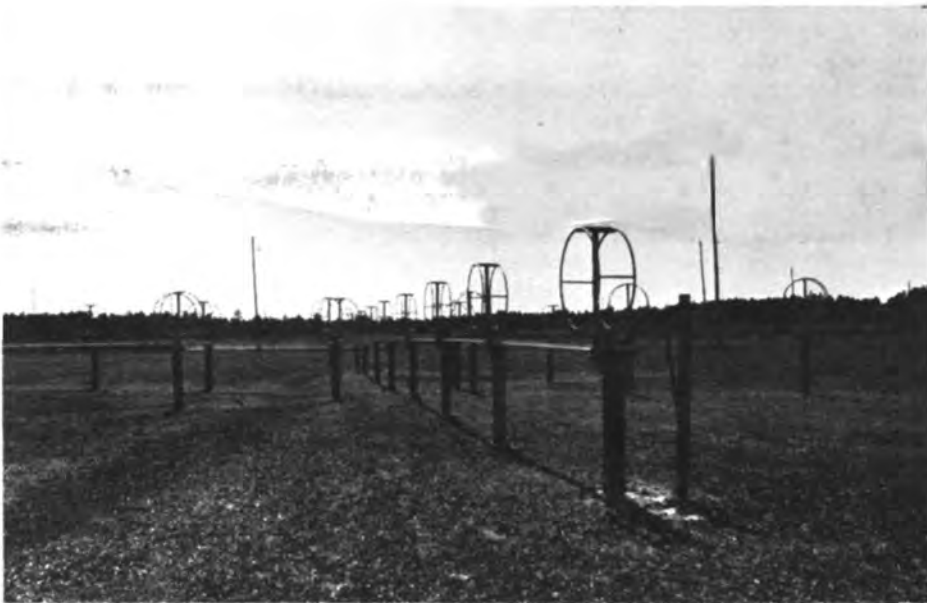
WNU Wide angle view of WNU's "Hermes" Directions" - Omni Directional receiving antenna array.
